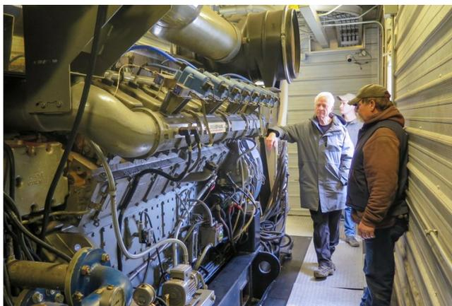
*Eric Edwards, right, Tom Vessels and Eugene Vessels, in rear, inspect one of the generators at the Elk Creek mine on Wednesday, March 17, 2021. The generator uses the captured methane gas to create electricity which then goes into the power grid.*
